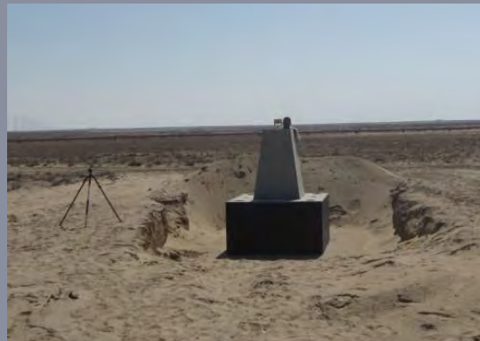
New pillars are 'surveyed into' same location.
