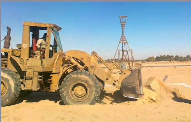
Old marker removed.
