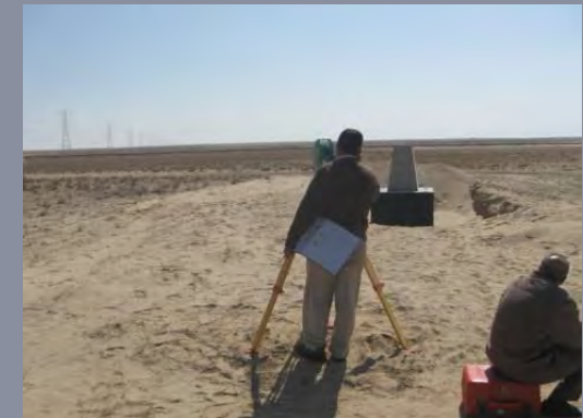
New pillars are 'surveyed into' same location.
