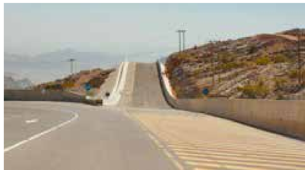
Safety Ramp, Jebel Akhdar, Oman
