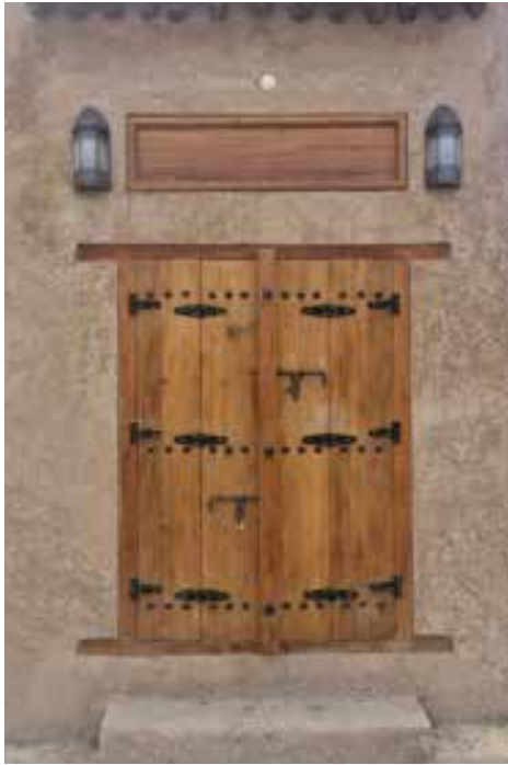
New doors in the Bahla Souq area, Oman
